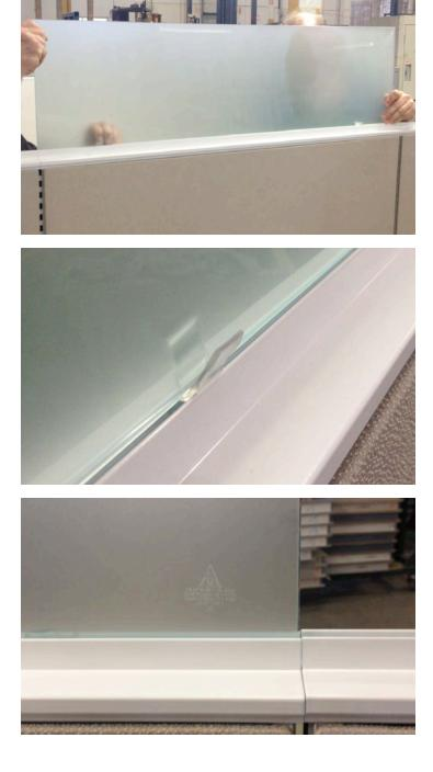
15. Ensure that the 2 adjacent privacy glass pieces are aligned and a tight gap is left between the 2 edges (3/32")
