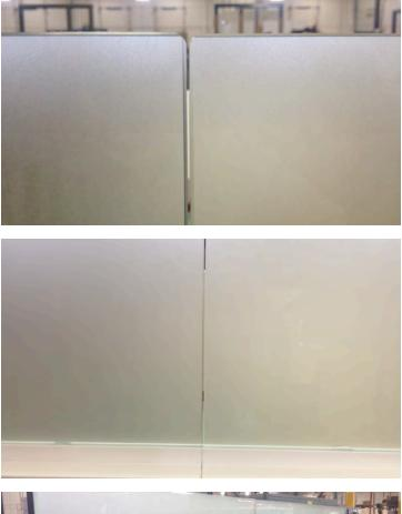
16. Installation of privacy glass is complete with shiny side out and log on the bottom left corner
