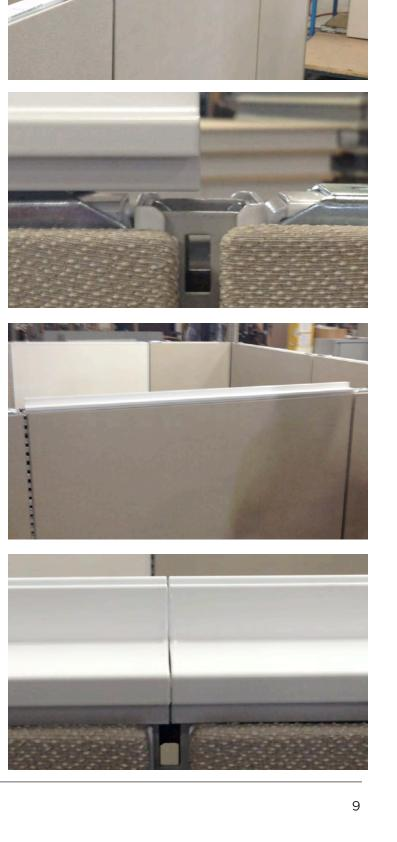
9. Plastic seal with grooves on the top side For ease of installation, use 1/2" plastic seal
