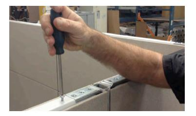
2. Install block and screw back using the same screw. It is important to start the installation from the middle panel.
